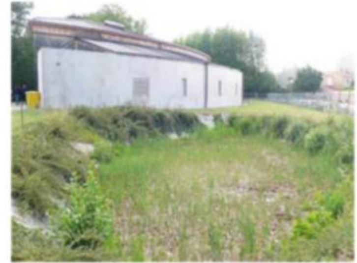
2. Infiltration basin (photo: K. Perini)
