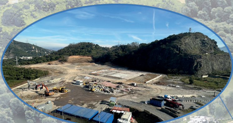
NEW POLYTECHNIC SCHOOL - Under construction Area equal to 60,000 sqm
